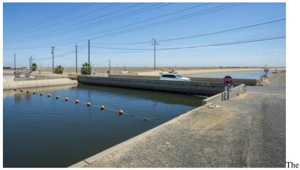
drought has caused a bridge over a Firebaugh, California, irrigation canal to subside until there's almost no space between bottom of bridge decking and canal water surface. (Florence Low/ California Department of Water Resources via AP)
